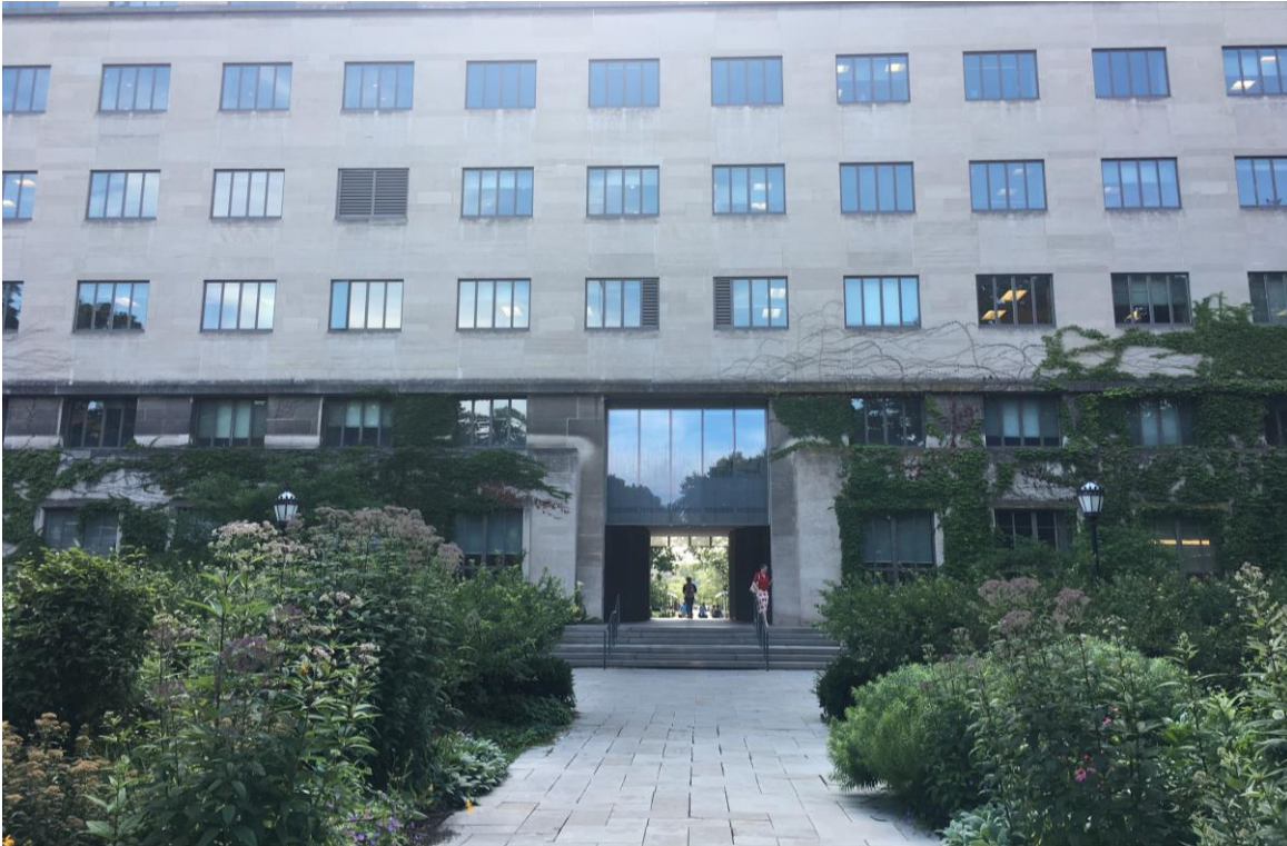
Edward H Levi Hall, connecting to the Main Quad
